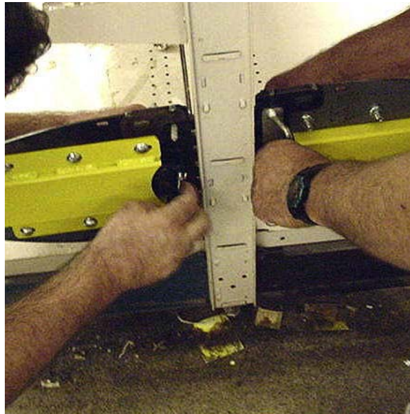
Lift Finger Installation
